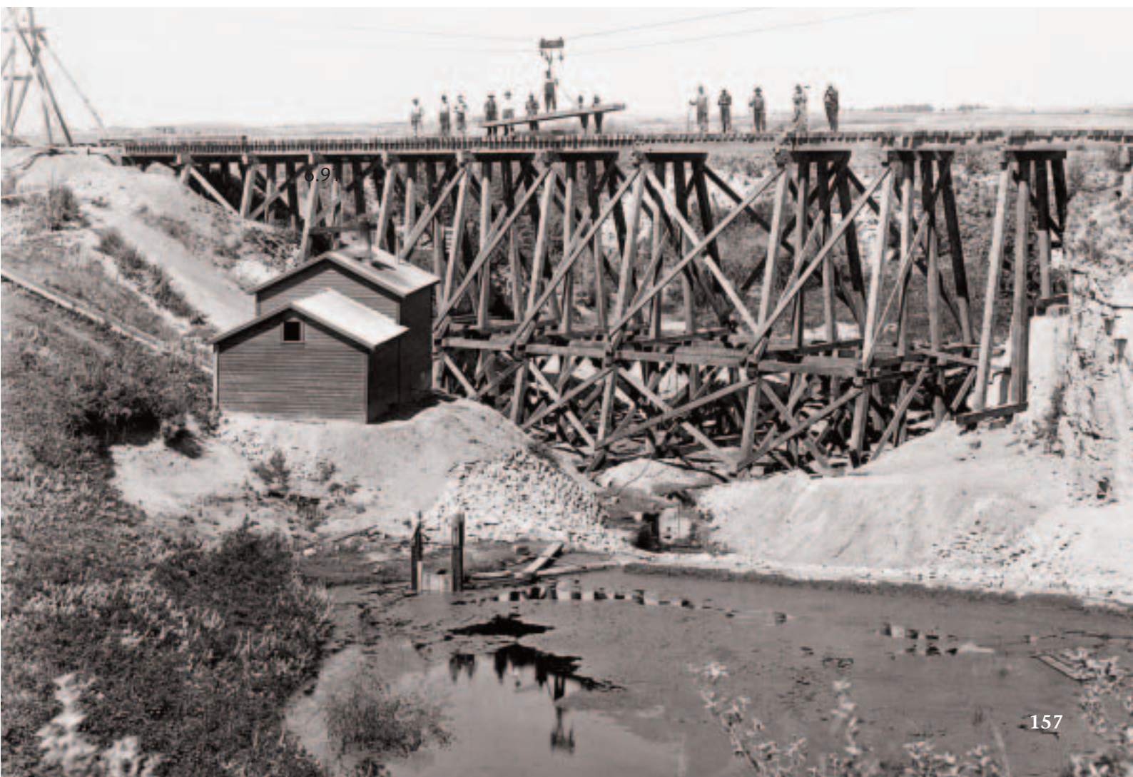
Building a railway bridge over Beaver Dam Creek, near Castor
