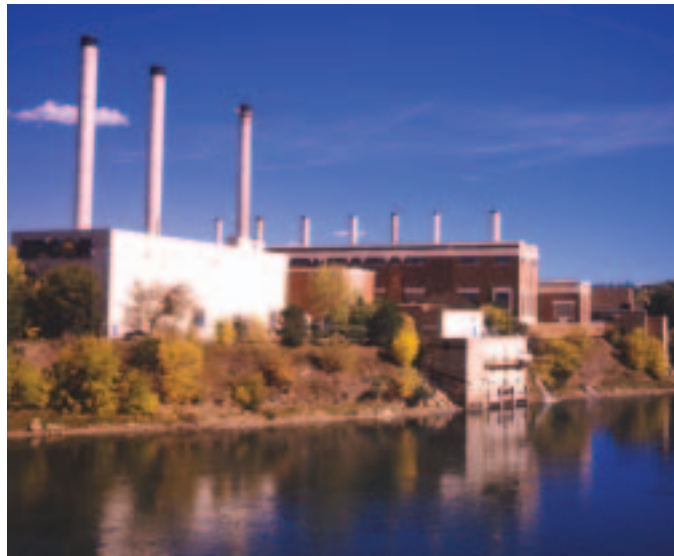
Rossdale Power Plant
